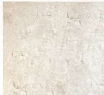
BBKR-8033 Shotcrete concrete
